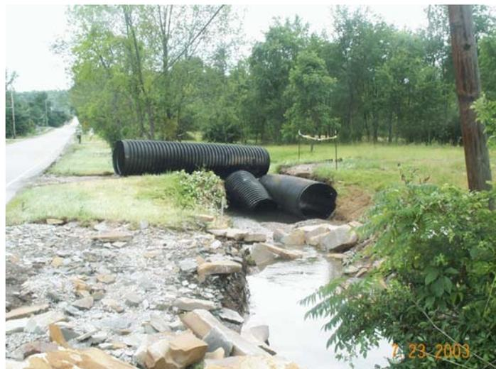
the last few years were able to withstand the torrential rains without washing out. But as stated earlier, unfortunately there were older drives with now under-sized culverts and some of these culvert pipes were just not able to withstand the additional waters.
